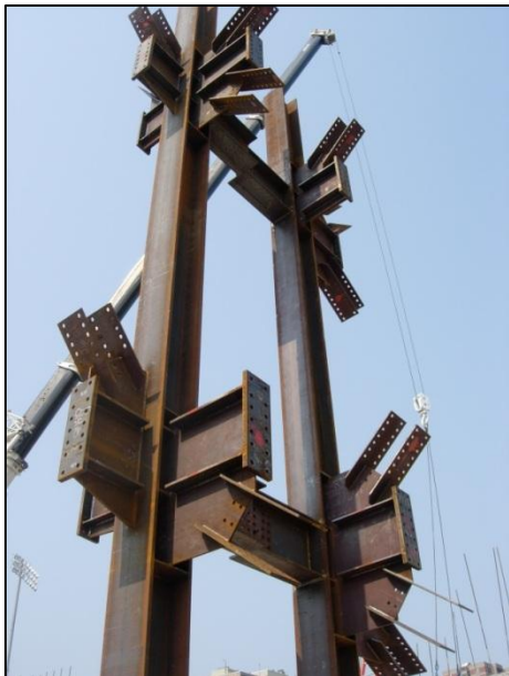
Figure 6: Connection construction photo
